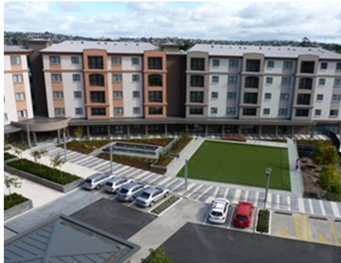
View of Metlifecare The Poynton Buildings 3 and 4 with croquet green
